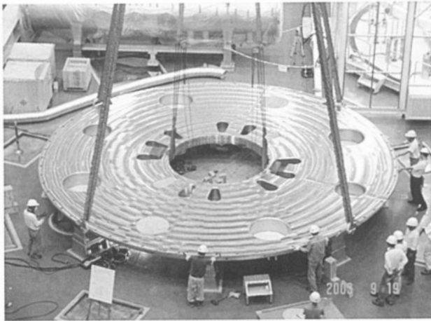
Fig.8 Movement of cryostat base plate on site (Sep. 2003)
